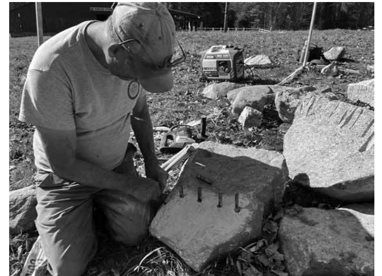
Mike Barwell. He's hiding his face, but it's no secret what Mike is up to; he's using feather and wedges to improve the face and sizes of large capstones and cornerstones.
