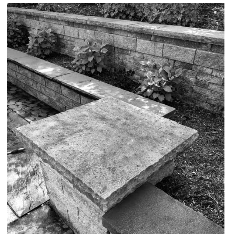
Pillar cap after cleaning with hot water pressure washer
