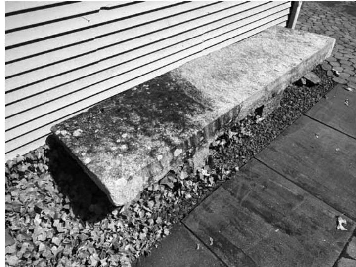
Granite bench left side not hot water pressure washed. Right side hot water pressure washed
