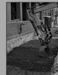
CU-STRUCTURAL SOIL® PORTSMOUTH
